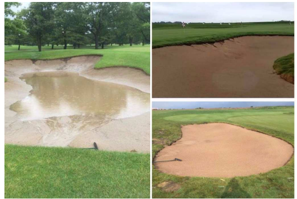
Pictures taken after 1.25 inches of rain. Image on left is our current on-course bunkers without an aggregate liner. Images on right are the newly constructed bunkers at MGTC with liners.
